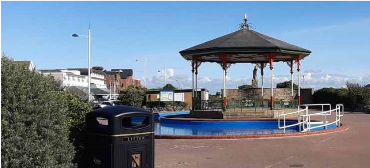
Plate 13 Bandstand Approximately 70 Metres Southeast of St Annes Pier
