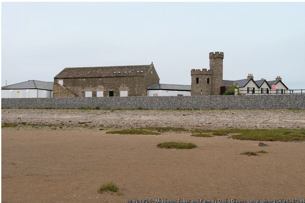
Plate 4 Olde Farmhouse, Middleton Tower Holiday Camp and Tower Approx. 10 Metres West of Ye Old Farmhouse
