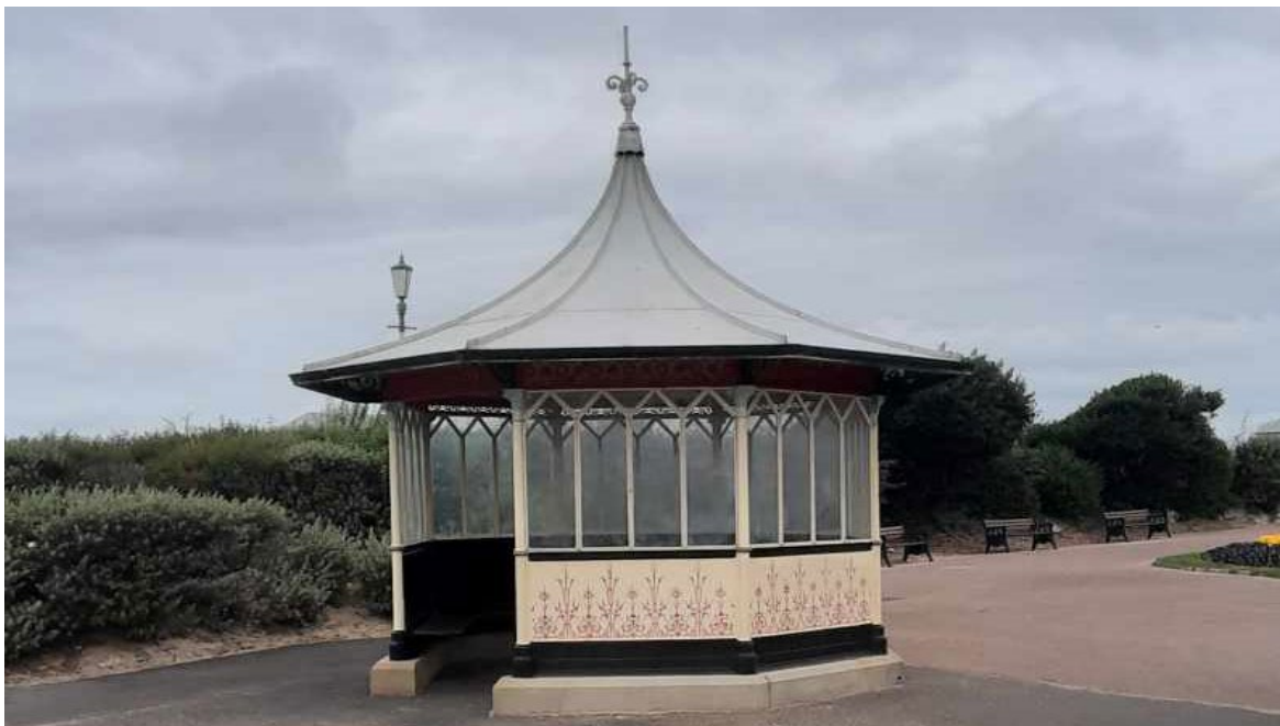
Plate 14 Octagonal Pavilion approximately 130 metres southeast St Annes Pier
